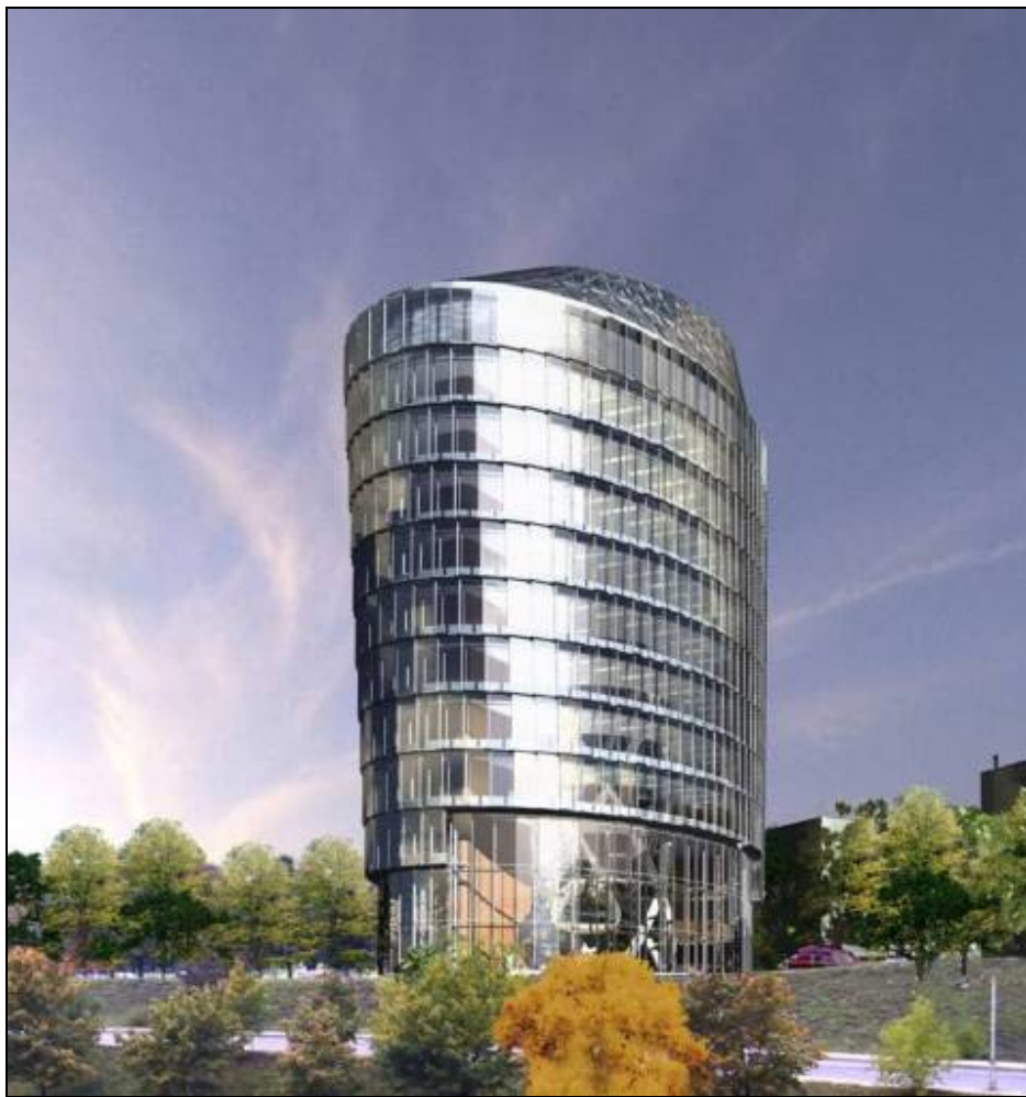
Fig 61: SBA Group new innovative office building (Vilnius, Lithuania)
